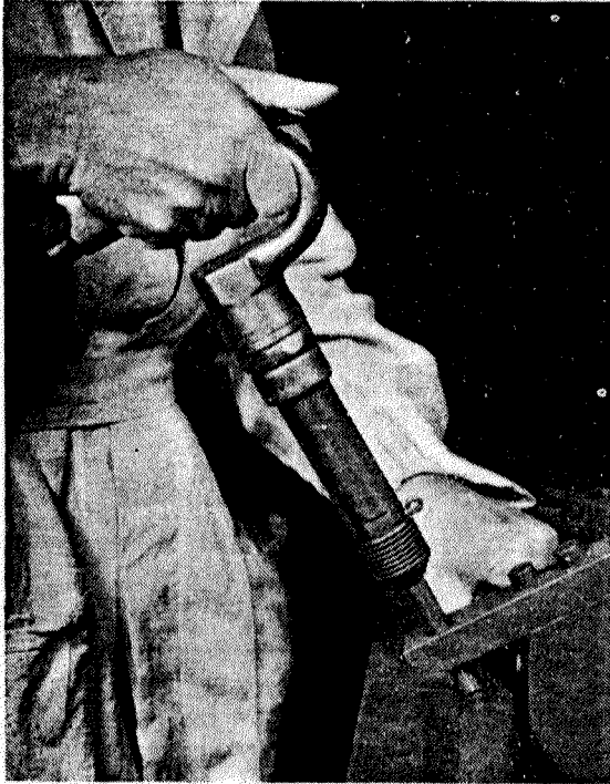
Fig. 9.9 Hammer peening a shaft.
