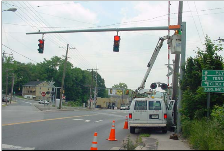
Figure 26. Inspection of a Mast Arm Structure.
