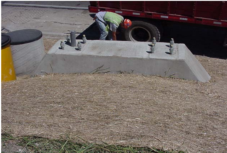
Figure 5. Foundation Ready for Structure Installation.
