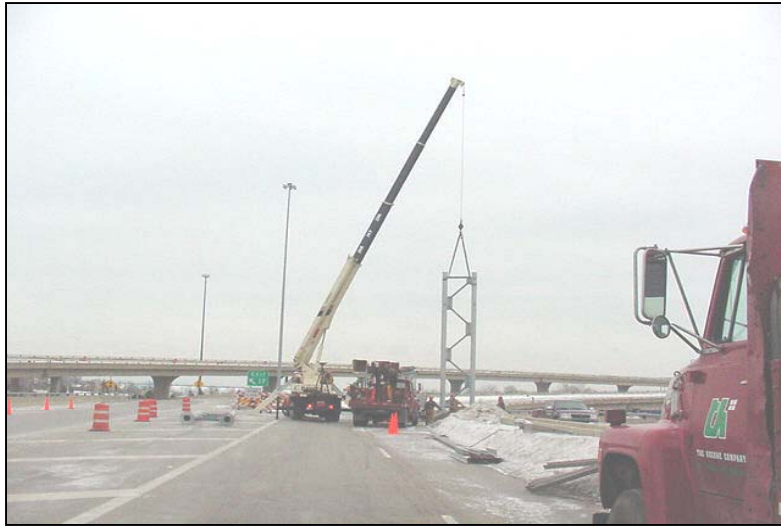
Figure 6. End Frame Being Set Onto Its Foundation.
