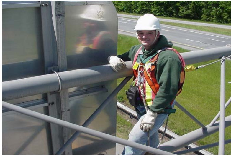
Figure 19. Inspector Uses Double Lanyard System.
