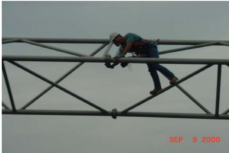
Figure 25. Hands on Inspection of Overhead Signs.
