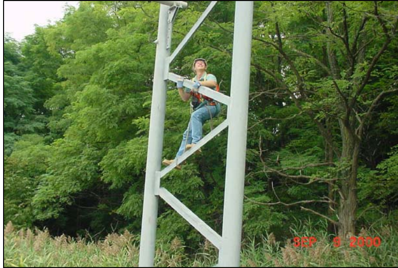
Figure 17. Inspector Climbing Structure.
