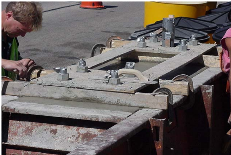
Figure 14. Template Secured to the Forms to Ensure Proper Alignment. Note Anchor Rod Threads Taped to Prevent Contamination by Concrete.
