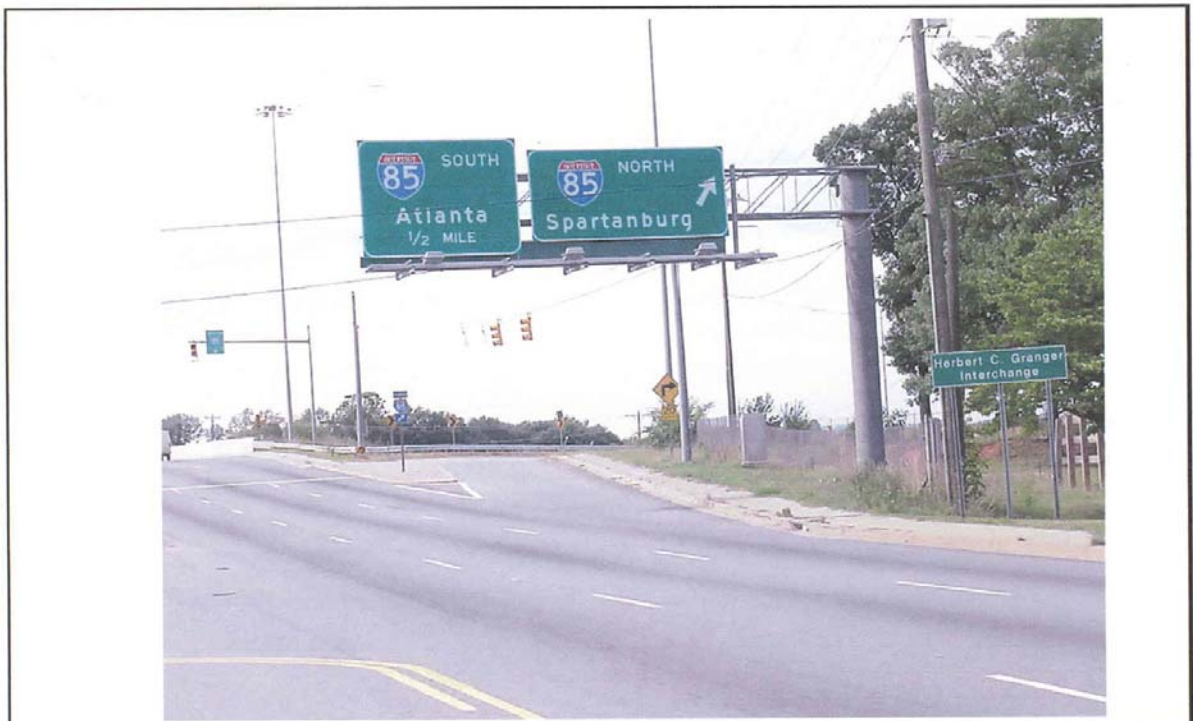
PHOTOGRAPH 1: FRONT OF STRUCTURE
