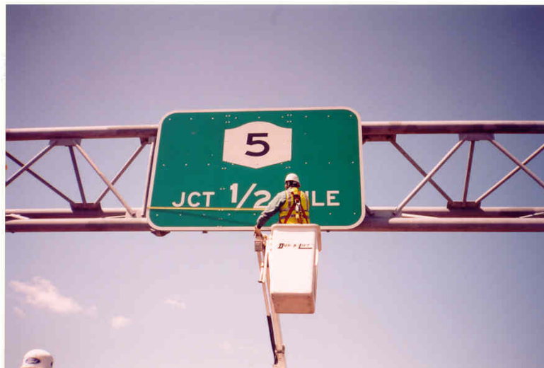
Figure 16. Inspector Measures Sign Panel During Inventory/Inspection Operation.
