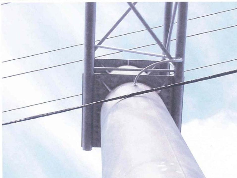
PHOTOGRAPH 4: COLUMN TO ARM CONNECTION
