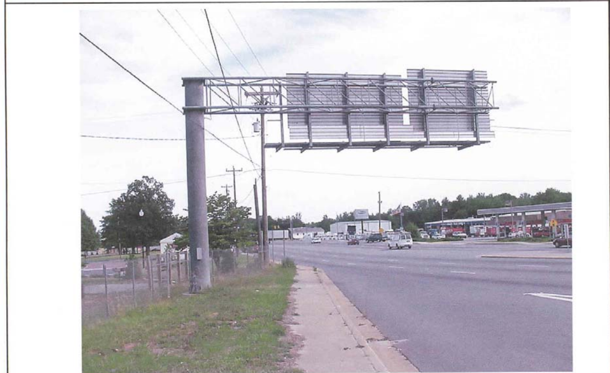
PHOTOGRAPH 2: BACK OF STRUCTURE
