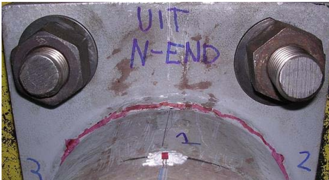
Figure 3.10 Highlighted Fatigue Crack on Specimen DU Mast Arm Weld Toe Along the UIT Application Line (90,680 cycles)
