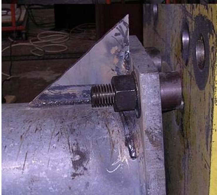
Figure 3.12 Stiffener Added to Mast Arm DU After 116,876 Cycles
