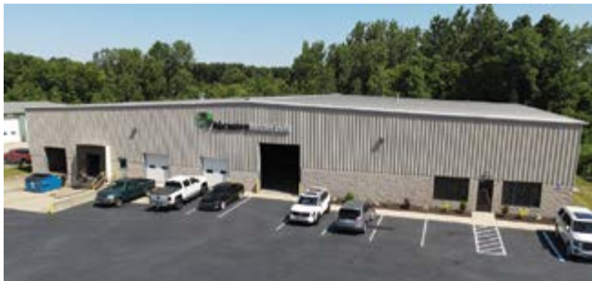
Abrasive Materials’ new location in Battle Creek, Michigan allows for additional inventory, increased production, and more space for lab facilities.
