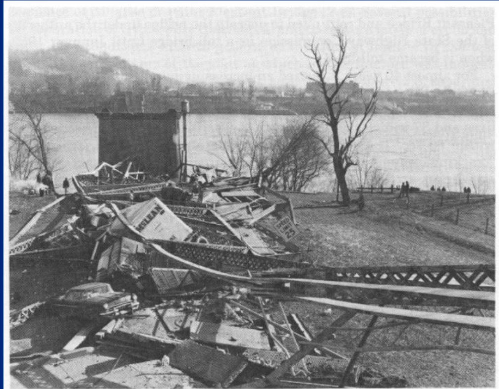
Figure 2.6 Point Pleasant Bridge after collapse (courtesy of Federal Highway Administration).
