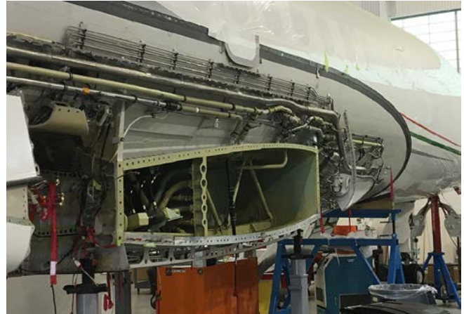
Figure 1: On-site shot peening of aircraft
