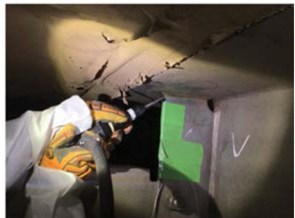
Fig.7 Crack closure treatment status
