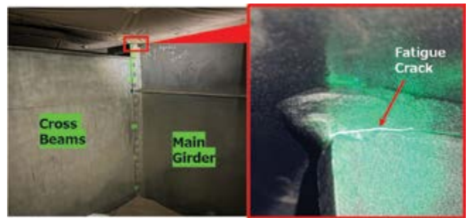
Fig.3(b) Fatigue crack (main girders with cross beams)
