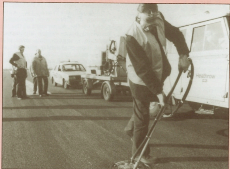
Two views of the Vacu-Blast runway light cleaner in operation.
