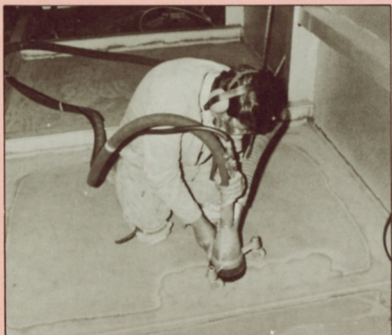
Working with a Closed-Circuit machine inside a steel box girder on the Tay Road Bridge.
