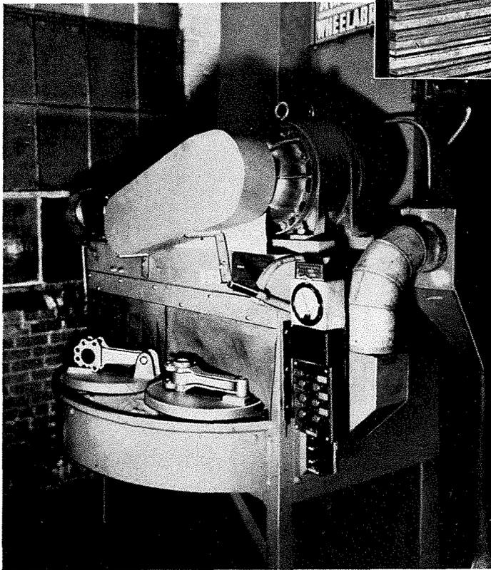
This No. 1 Wheelabrator Table is used for Wheelapeening (cold working to increase fatigue life) aircraft master connecting rods at Jacobs Aircraft Engine Co., Pottstown, Pa.
